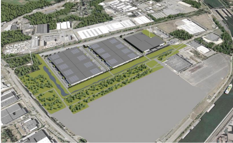
Genk Green Logistics Redevelopment zone B
